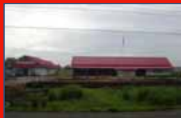
District office of Fire brigade, Kallier
