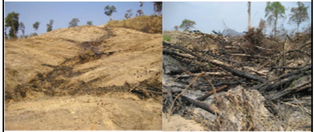
Pushing debris or soil into drainage lines
