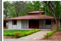
Two bedroom guest house at IPIRTI campus
