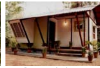
Demonstration house at IPIRTI campus
