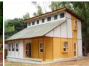
Two storied bamboo house built at IPIRTI campus
