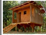
Prefabricated BMB- wood shelter at IPIRTI campus
